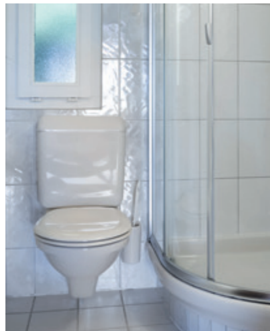
BEFORE Installation situation with exposed cistern
