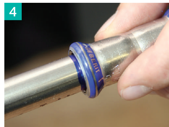
INSERT PIPE INTO FITTING
