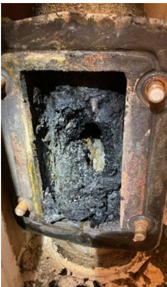
An opened cleaning eye reveals a thick layer of congealed waste inside
